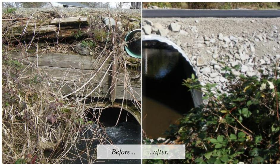
The project was located where Badger Creek passes under the Springwater Trail. The barrier "culvert" under the Trail—actually a set of three rusty and clogged culverts—was replaced with a single, large culvert that should not clog easily. Now fish and wildlife can move freely up and downstream at the site, and can access the 1.6 miles of upstream Badger Creek habitat.
