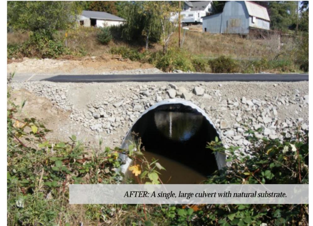
AFTER: A single, large culvert with natural substrate.
